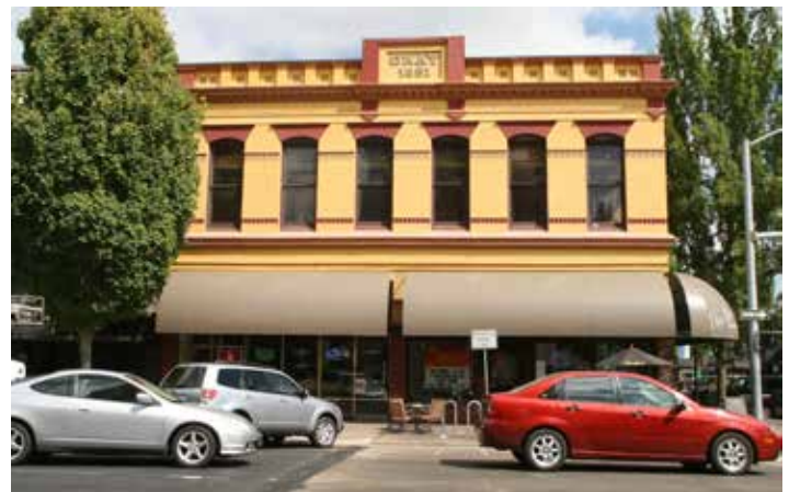
Photo: Courtesy of Heritage Consulting Group The Gray Building in Salem, Ore. is being rehabilitated with support from the 20 percent HTC and Oregon Special Assessment for Historic Properties.
