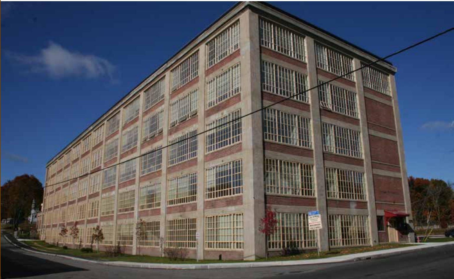
PMC Properties adapted the Dennison Manufacturing Company Paper Box Factory into 93 market rate apartments in Marlborough, Mass.
