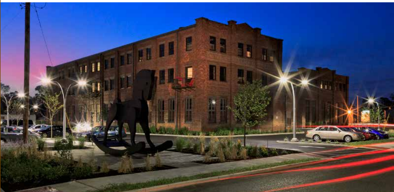
Lace Mill in Kingston, N.Y., recently completed its rehabilitation, which included the construction of an addition.
