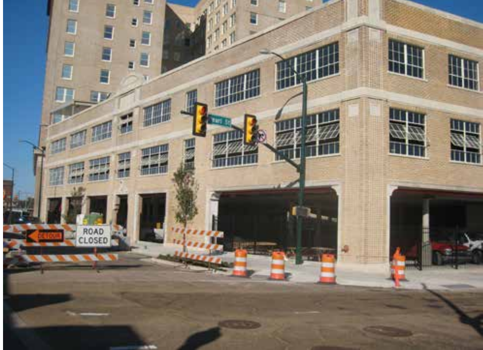
Image: Courtesy of Heritage Consulting Group
