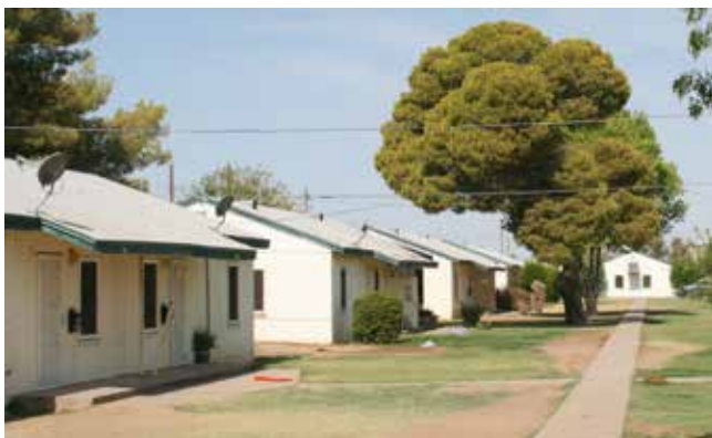
Photo: Courtesy of Heritage Consulting Group Gorman & Company's rehabilitation of Coffelt Lamoreaux public housing will create fresh affordable housing units in Phoenix, Ariz.
