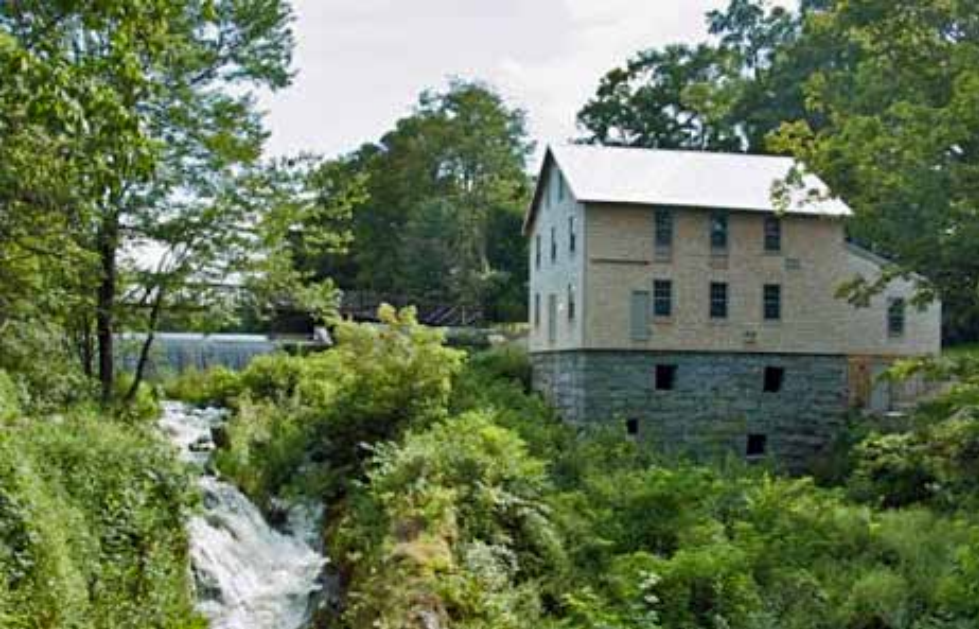
Image: Courtesy of Courtesy of Heritage Consulting Group The Mill at Freedom Falls in Freedom, Maine, will install a 50kW turbine this fall that should produce 70,000 kWh or power annually.
