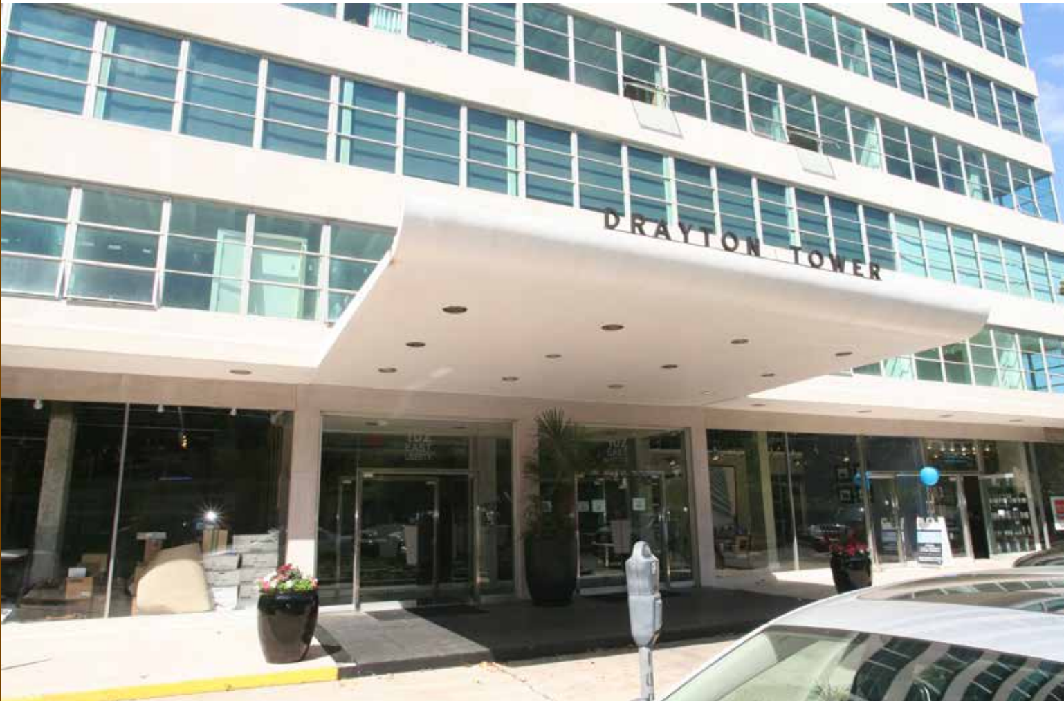
Image: Courtesy of Heritage Consulting Group Drayton Tower in Savannah, Ga., was rehabilitated by Flank, a New York City-based developer, using historic tax credit equity.
