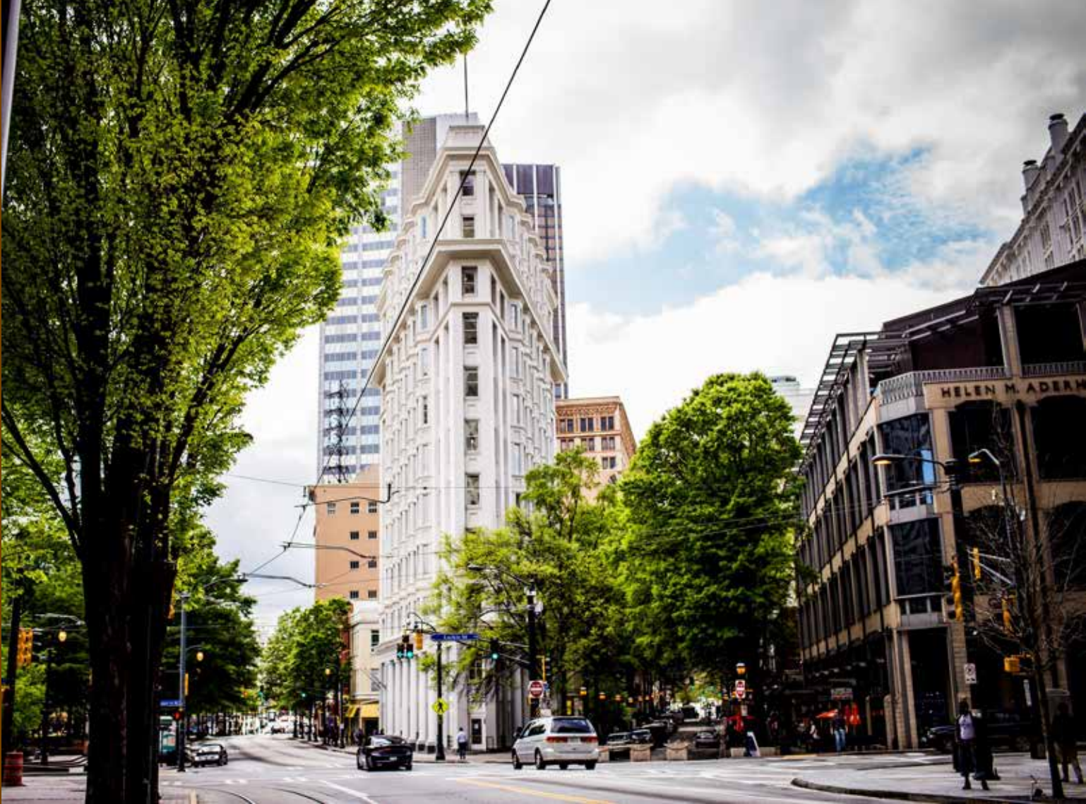
Image: Courtesy of Heritage Consulting Group
