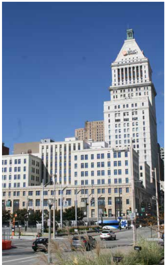
Image: Courtesy of Heritage Consulting Group The Union Central Life Insurance Company Annex in downtown Cincinnati was preserved using the Ohio State Historic Preservation Tax Credit and the federal historic tax credit.
